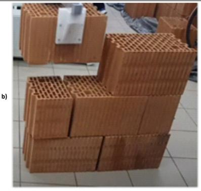
Fig. 14.b View of the bricklaying process on a partition wall: lay bricks on the wall  $\left[ 16 \right]$
