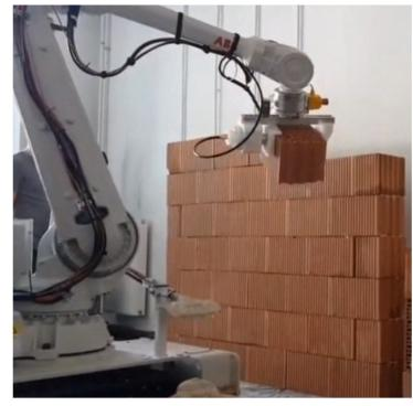
Fig. 14.a View of the bricklaying process on a partition wall: industry robot while bricklaying [16]
