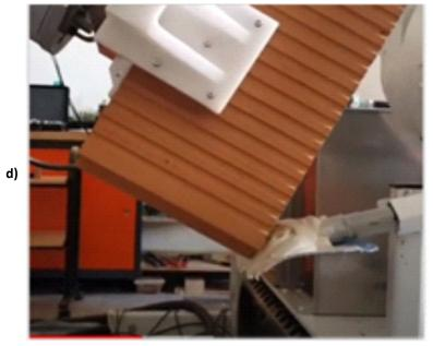
Fig. 14.d View of the bricklaying process on a partition wall: apply mortar to the bricks [16]
